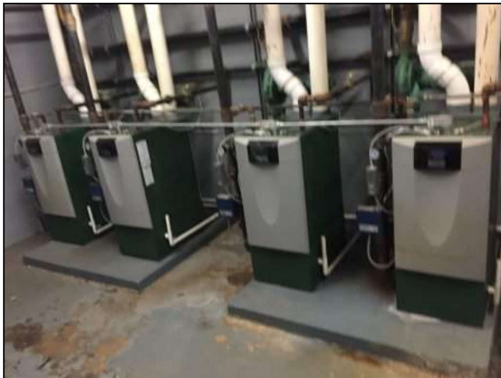
Building 7 Gas Fired Heaters
