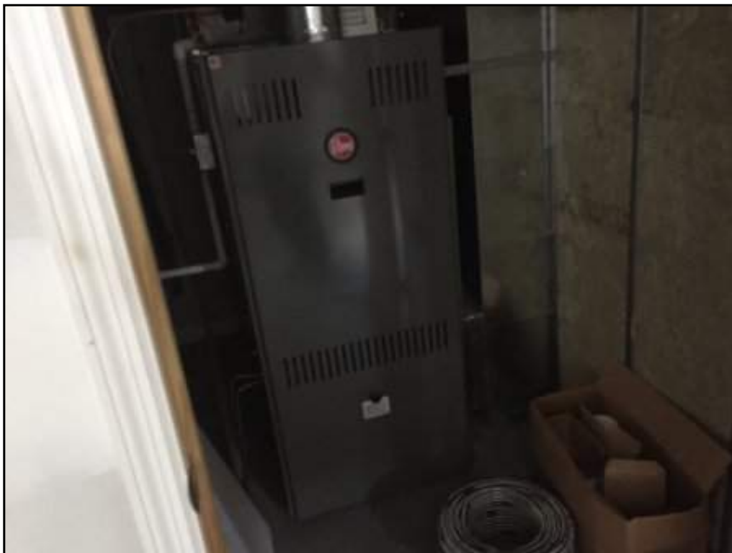
Single Unit Oil Fired Heating System (typ.)
