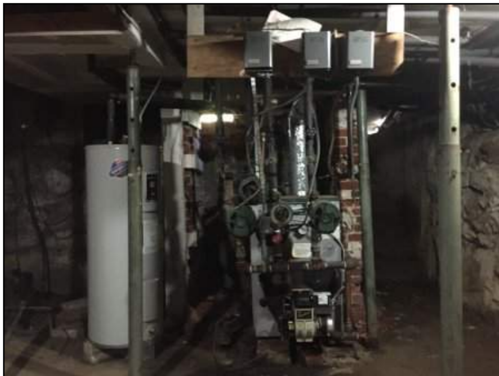
House B Oil Fired Heating System (Basement)
