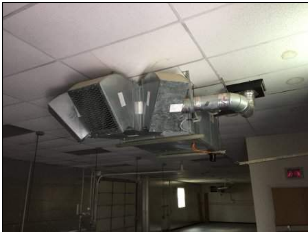
Single Unit Oil Fired Heating System (typ.)
