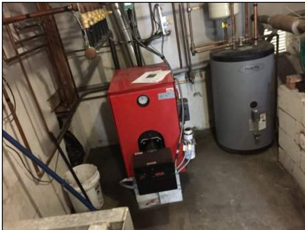
House B Oil Fired Heating System (Garage)
