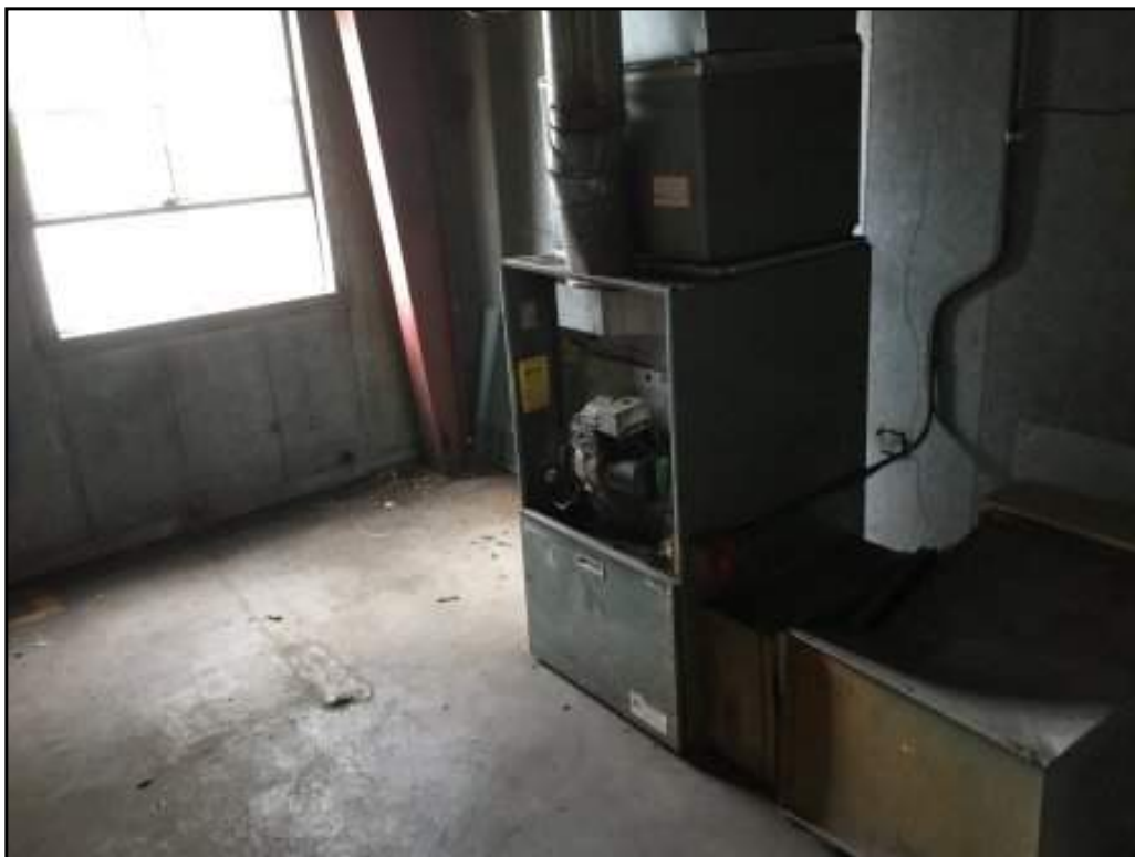
Single Unit Oil Fired Heating System (typ.)
