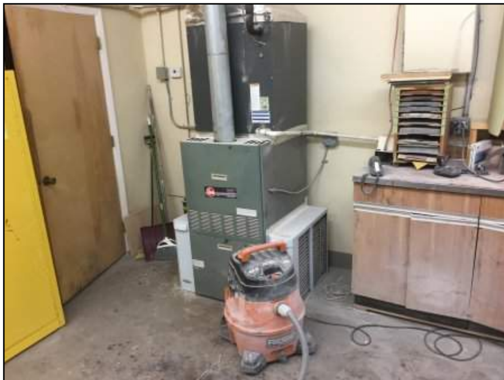
Single Unit Oil Fired Heating System (typ.)
