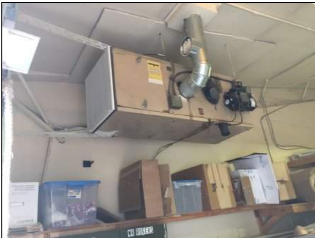
Single Unit Oil Fired Heating System (typ.)
