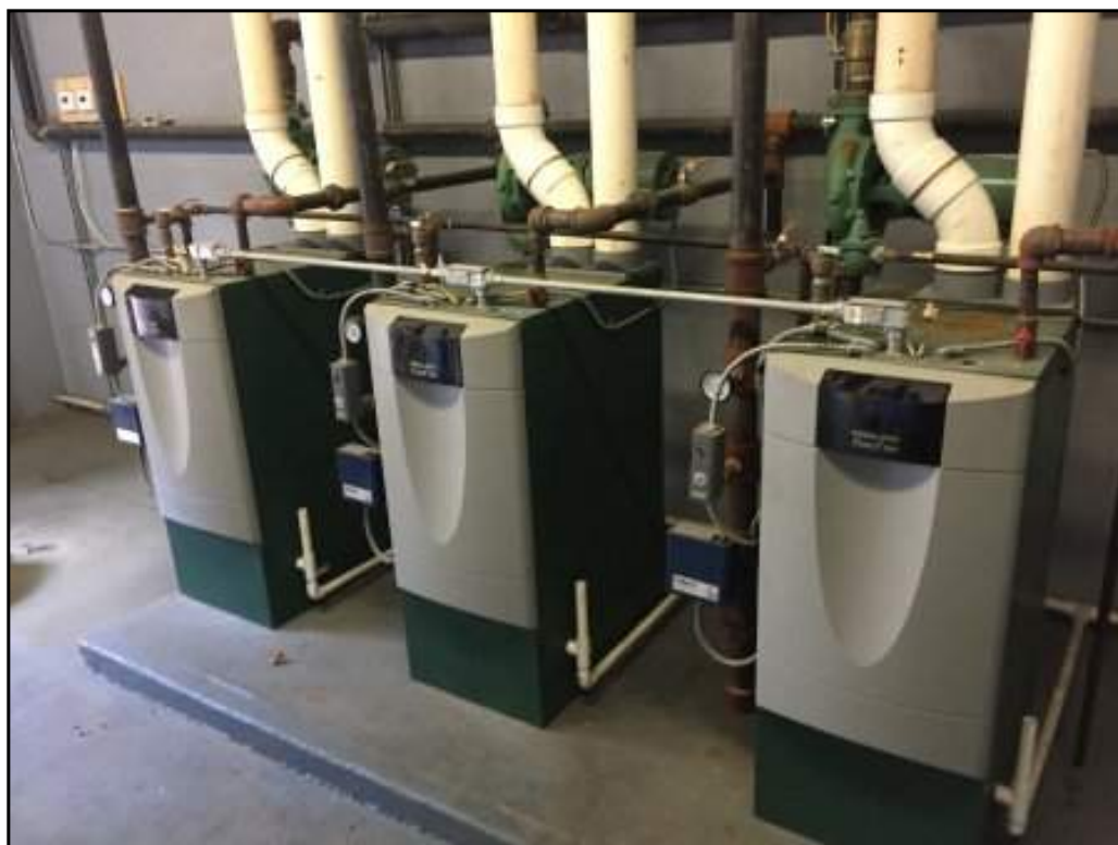
Building 7 Gas Fired Heaters
