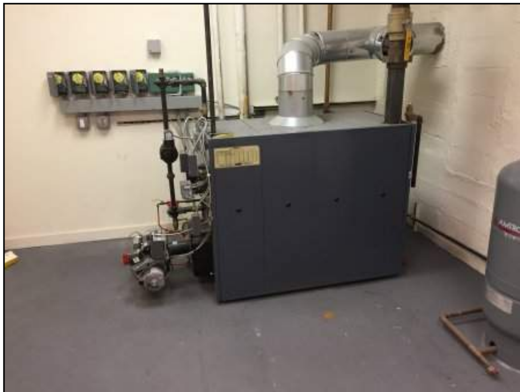
Building 1 Oil Fired Heater
