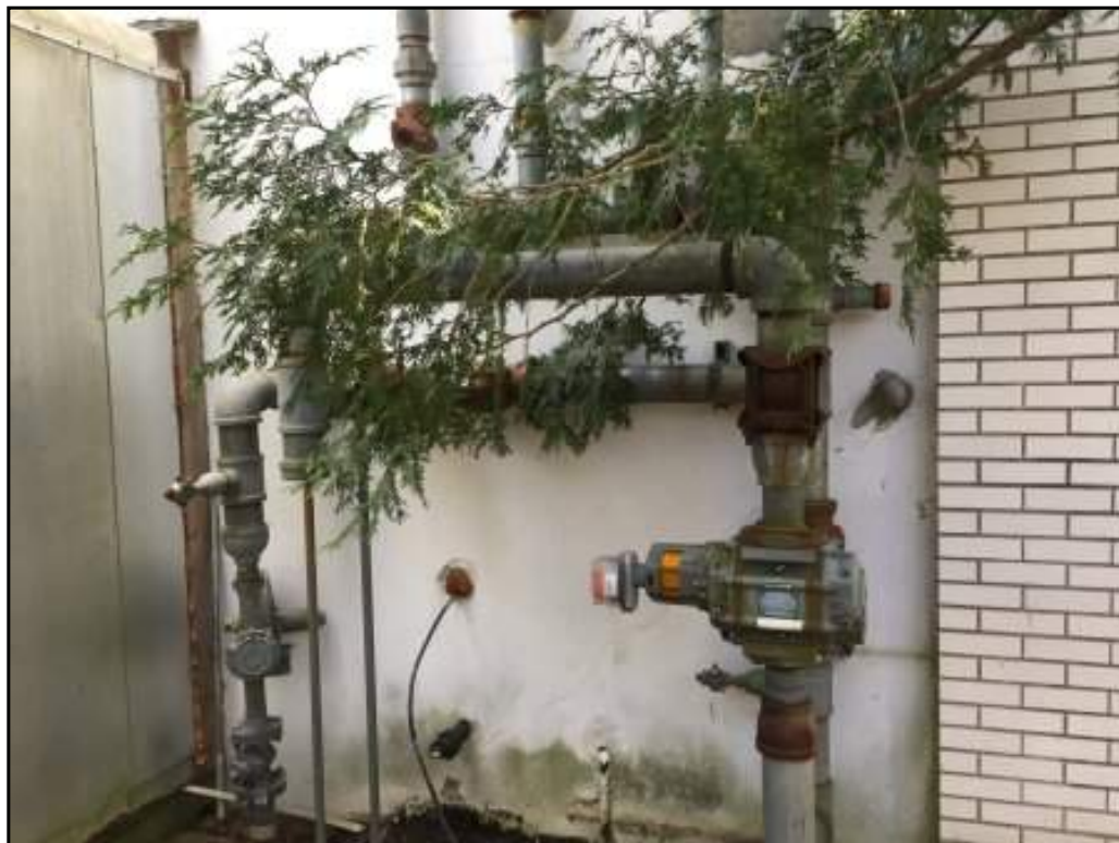
Catering Facility Gas Meter
